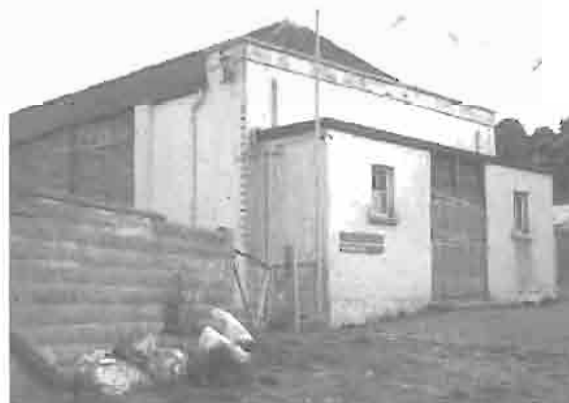
St. Dogmaels Memorial Hall before renovation work began.
